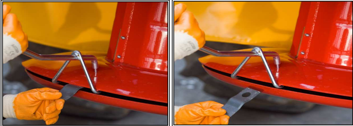
Pic.16- Replacing the knives
